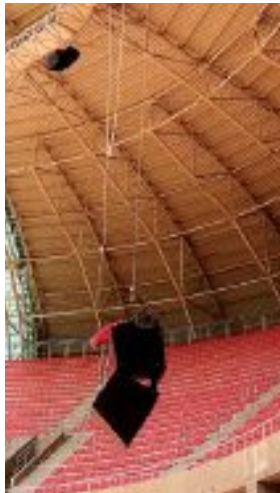
Each hang was winched into place; APCO also took on the PA/VA solution for the stadium
